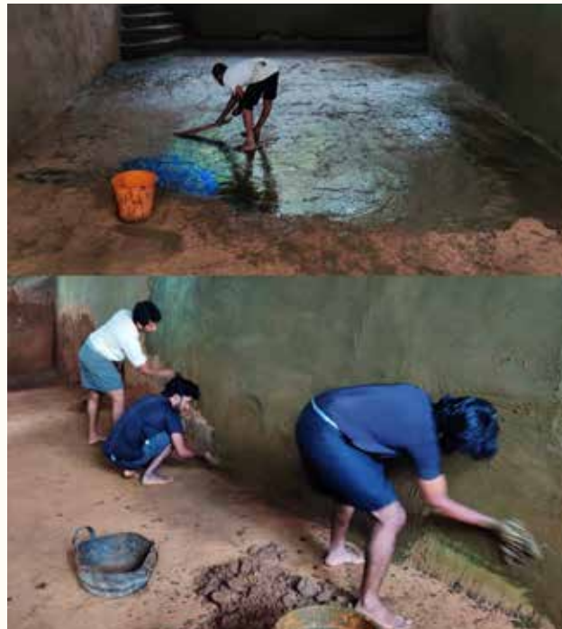
Volunteers Amal, Ali, and James assist Sudhi in repairing the barn
